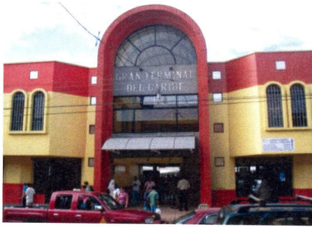
Fig. 35. Bus Terminal, Port of Limón
